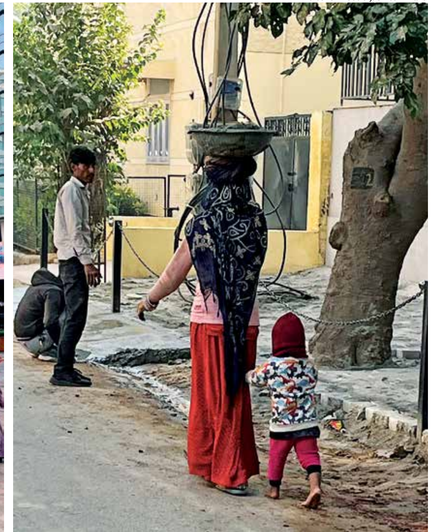
And a women labourer with her child at a construction site
