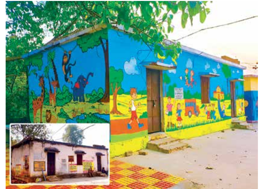
Before and after: In Odisha, the Jaga Mission provides all facilities
