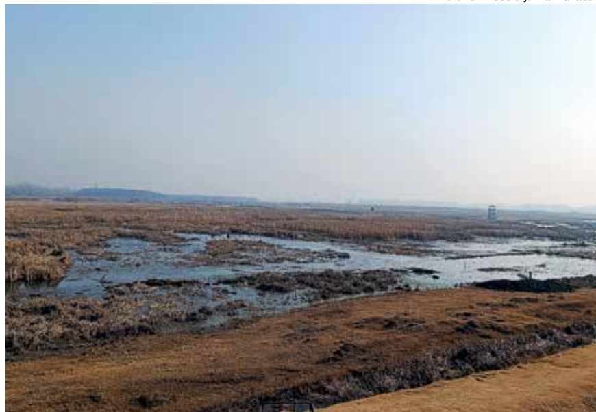
The Shallabugh wetland where there have been five breaches
