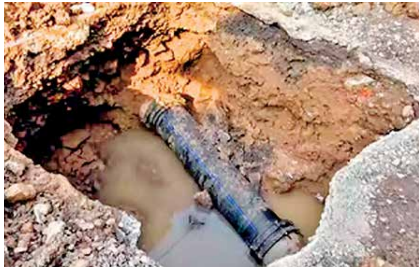
Pipelines have to navigate through dense settlements, sewage lines and drainage systems
